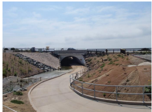
Access to Moro beach from campground, under PCH
